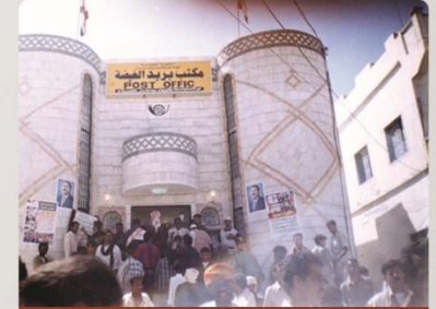
Ghaidha Post Office Construction
