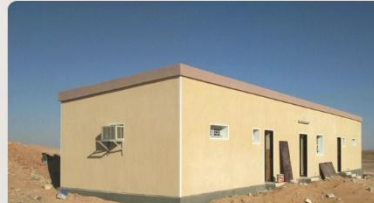
Godah DNO Construction Project
