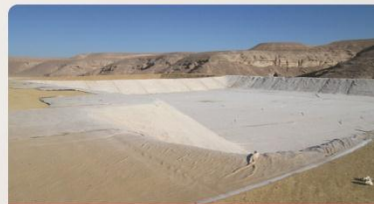
Dhahban Well Platform
