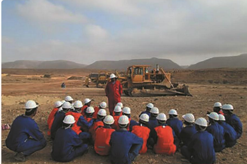
Environmental Cleanin Project at MOL K55
