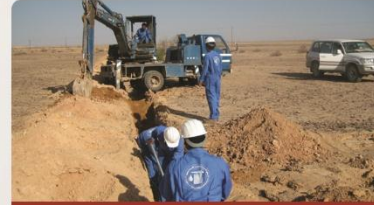
Pipe Line Project
